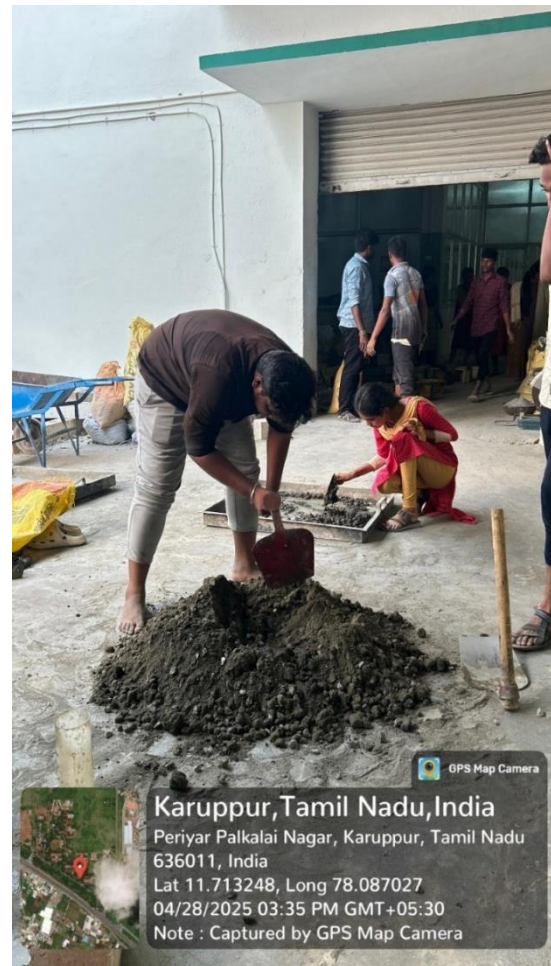
Fig.6 Mixing Of Concrete
