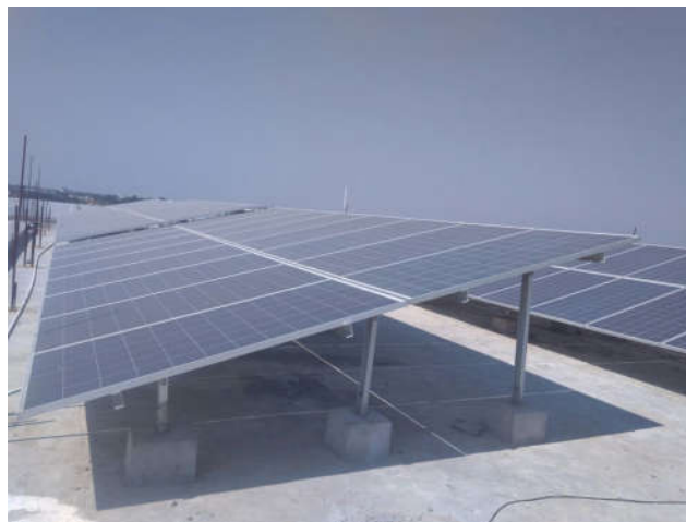
Fig.5 Actual onsite of 80KW solar roof top PV modules at St.Peter's Engineering College, Hyderabad City
