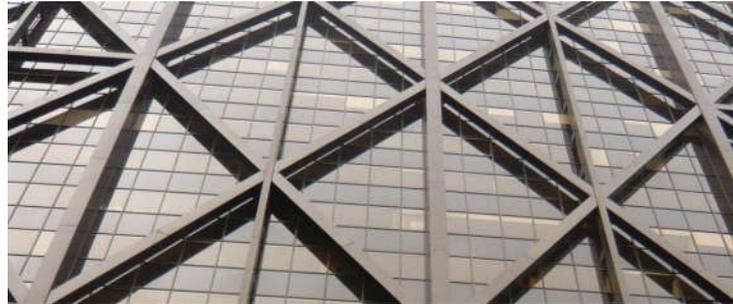
Fig. 8 X- bracing system [8]
